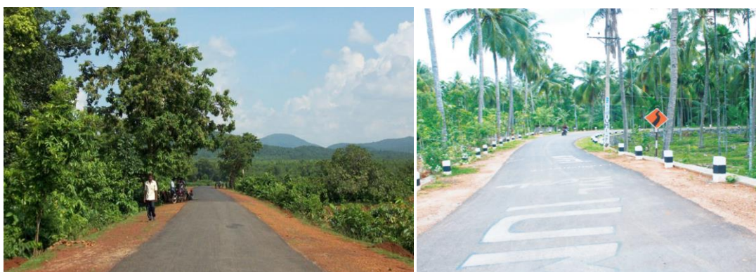
Fig. 14.5: Photographs showing well maintained shoulders for pedestrians to Walk
